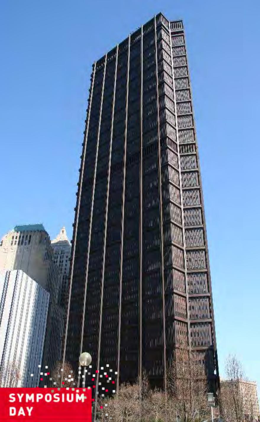
*It was the first structure in the nation to use liquid-filled, fireproofed columns as a safety feature. The 18 support columns are filled with a mixture of water and anti-freeze. It was the best the steel industry could produce, remaking the Pittsburgh skyline and towering over the city landscape*
